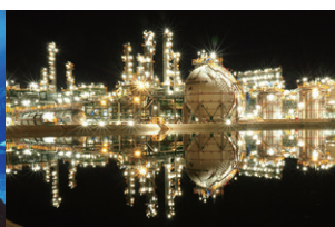
A plant in Thailand where Sumitomo Chemical licensed its propylene oxide production method
