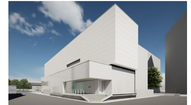
S-RAMCO Line 2 (under construction)
