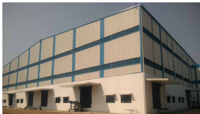
Vapi Plant, Sumitomo Chemical India
