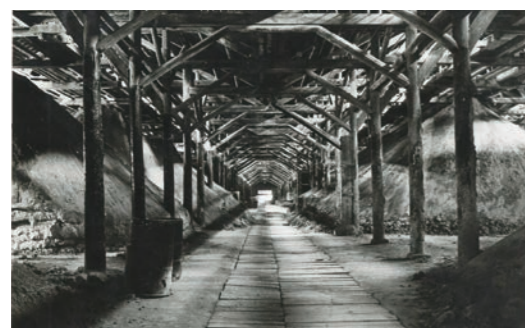
Calcium superphosphate warehouse
