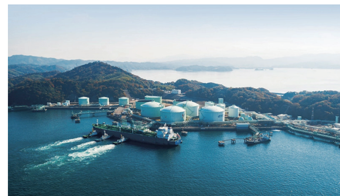
The existing terminal operated by Namikata Terminal Co., Ltd. (Imabari City, Ehime Prefecture)
