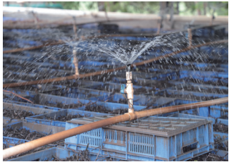
Water Treatment at the Bhavnagar Plant
