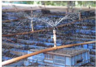
Water Treatment at the Bhavnagar Plant
